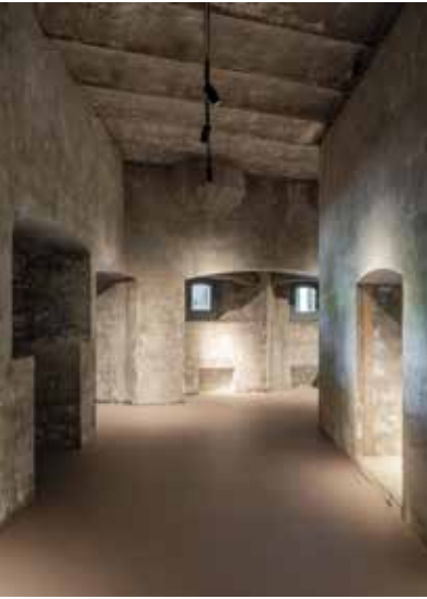
■ This page. Left: the staircase connecting to the underground postern corridors, which have been partly excavated for reuse. Two central photos: the fortified ground-floor chamber. It has been completely stripped and sandblasted to highlight the tactile and sculptural qualities of the concrete; it is now fitted with underfloor heating and the gun emplacements have double glazing. Right: the corridor connecting all the ground-floor rooms, which are now used as studios for creatives. Opposite page, from top: the area that housed the guns, now an exhibition space; view of the postern, connecting the main building to the upper courtyard
